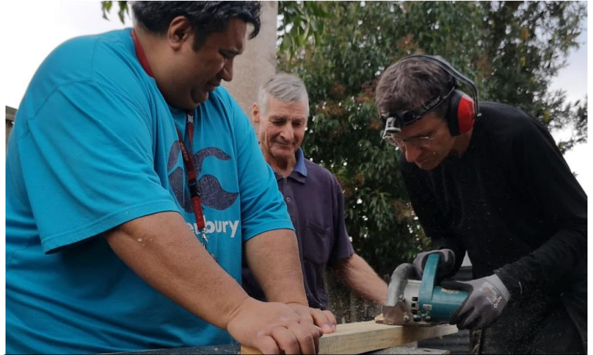
14 May 2020 - Bro Des, Bro Neville, Bro Steen, work together to help build a technician desk in the recording room.
